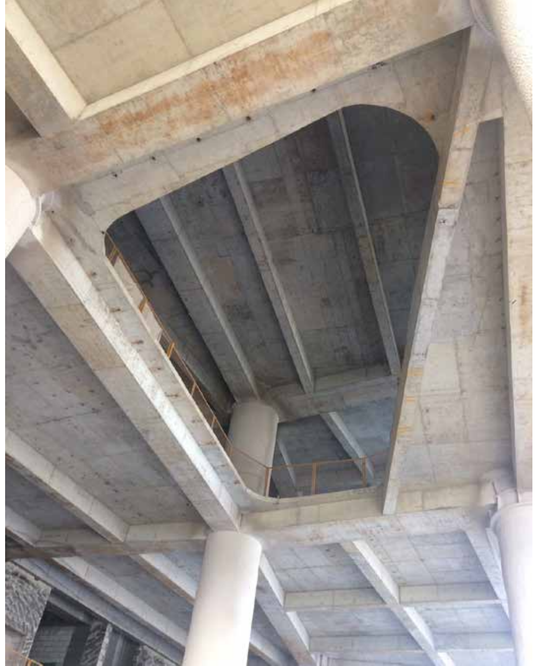
MAIN LOBBY AND GROUND FLOOR OF THE TOWER UNDER CONSTRUCTION
